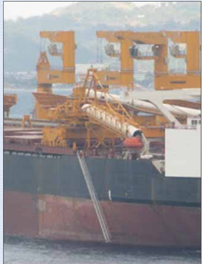
Ship Loader with transfer conveyors
